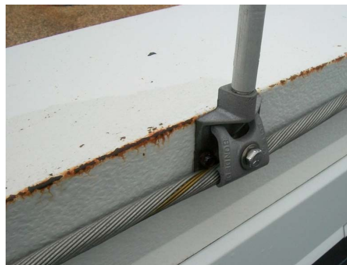
Figure 7: Aluminum side-mounted on painted steel.
