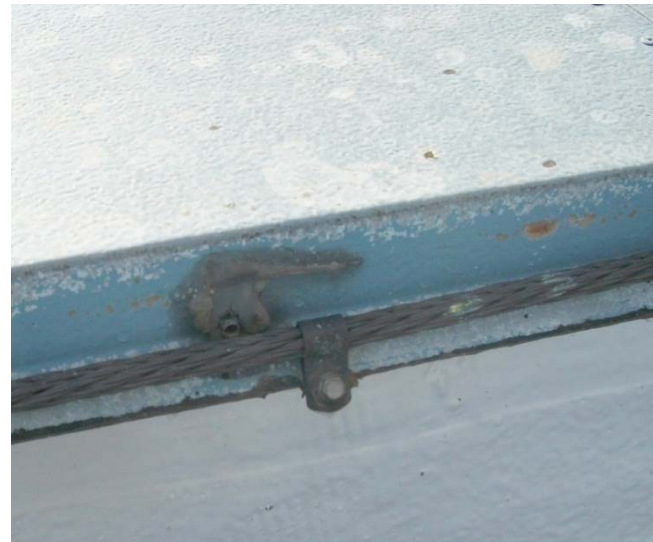
Figure 6: Copper side-mounted on painted steel.
