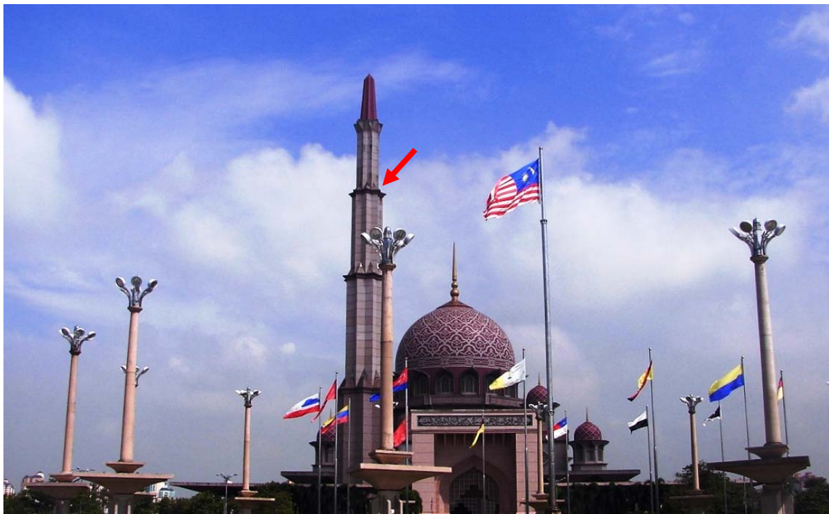
Figure 5: The arrow points to the location of the lightning damage in the 2005 incident.
