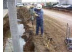
The most commonly employed grounding application utilizes ground rods composed of copper, copper-clad steel or stainless steel. These rods must extend vertically at least 3 meters (10 feet) into the earth. Factors such as soil content, environmental challenges and structural characteristics can dictate special grounding requirements or applications.
